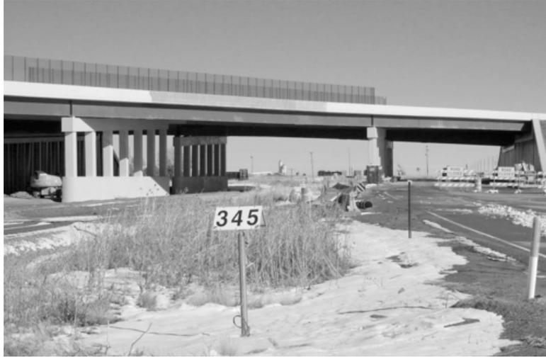
FIGURE 10. New triple-span bridge on I-70 over the transcontinental railroad near Denver's airport. The east end (right) is supported by reinforced soil. Pipeline marker is in foreground.
